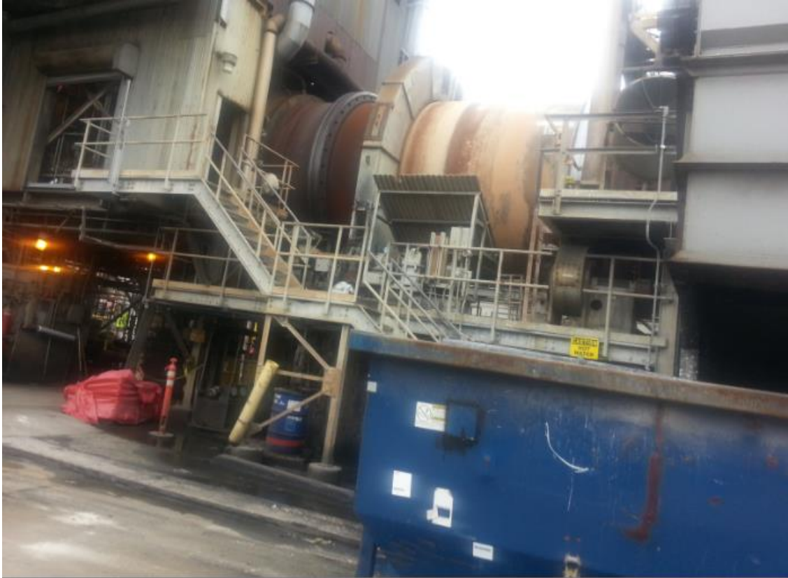
Figure 16 Train 1 with 3.6 Meter Diameter Kiln
